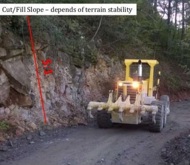
Cut/Fill Slope - depends of terrain stability
